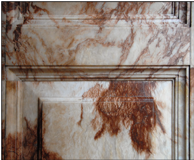
Figure 5. A small part of the second-floor doorcase made of alabaster from Tutbury.
