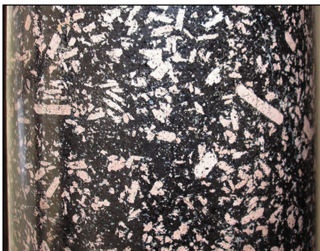
Figure 12. The luxullianite column in the Grotto, with its feldspars in a matrix of black tourmaline.
